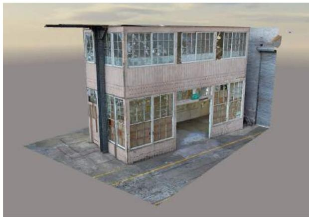
This part of the workshop was a “building within a building”. This originally was the foreman’s office for the maintenance teams. Pictured above is a colorized LiDAR point cloud. Image by Orion and Euclidean
